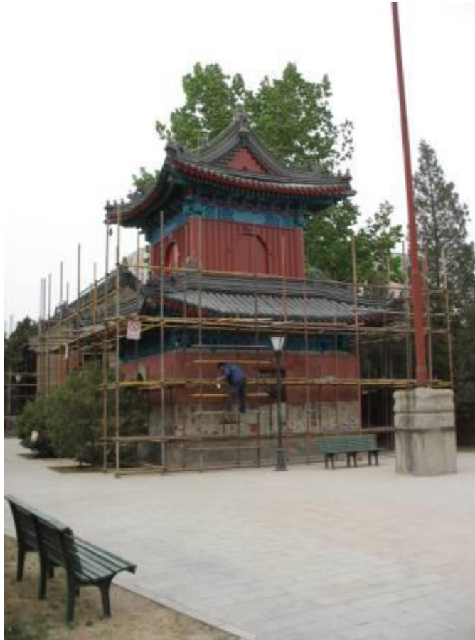
Restoring the Drum Museum, Beijing, 2006
