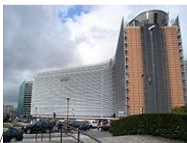
The headquarters of the European Commission, Brussels, Belgium
